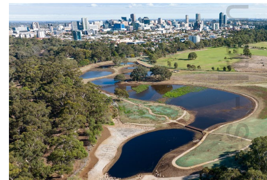
$13 million, 3.2 hectare wetland in the southern part of Victoria Park / Pakapakanthi (Park 16). The largest earthmoving exercise and redevelopment in our Park Lands in the past 60 years was a collaborative project with the Brownhill and Keswick Creeks Stormwater Board
